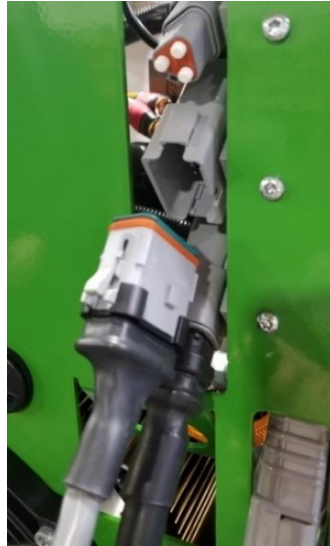
Figure 16. Disconnecting Controls Extension Harness
